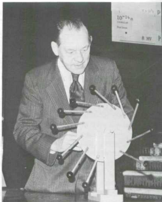
Plate 4.5 An alternative 'perpetual motion' machine that doesn't work either!
